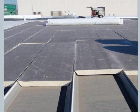
1. Fill the flutes with tapered insulation.
